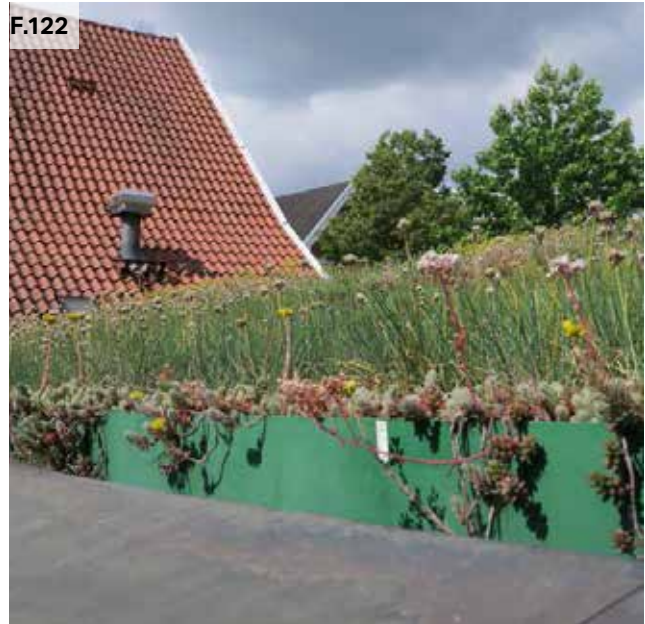
Figure 122: Detail of a green roof integrated into the fabric of the historic town of Rheda-Wiedenbrück, Germany.
