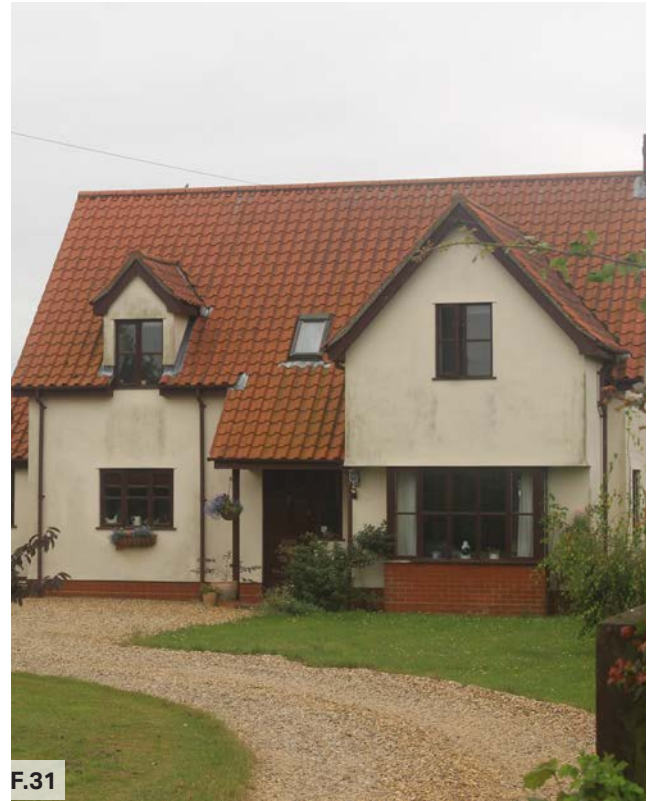
Figure 31: Development should respect the building setback from road and plot patterns providing front and back gardens.
