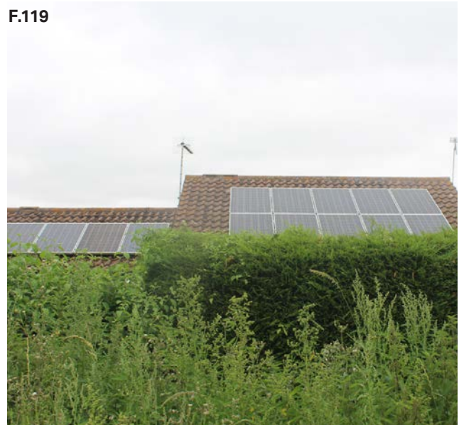
Figure 119: Solar panels installed on the south-facing pane of the roof of new build house in Wetheringsett
