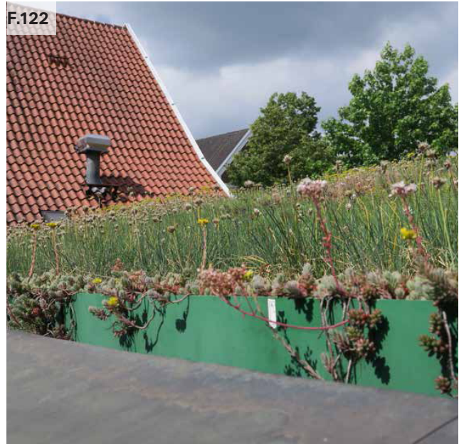
Figure 122: Detail of a green roof integrated into the fabric of the historic town of Rheda-Wiedenbrück, Germany.
